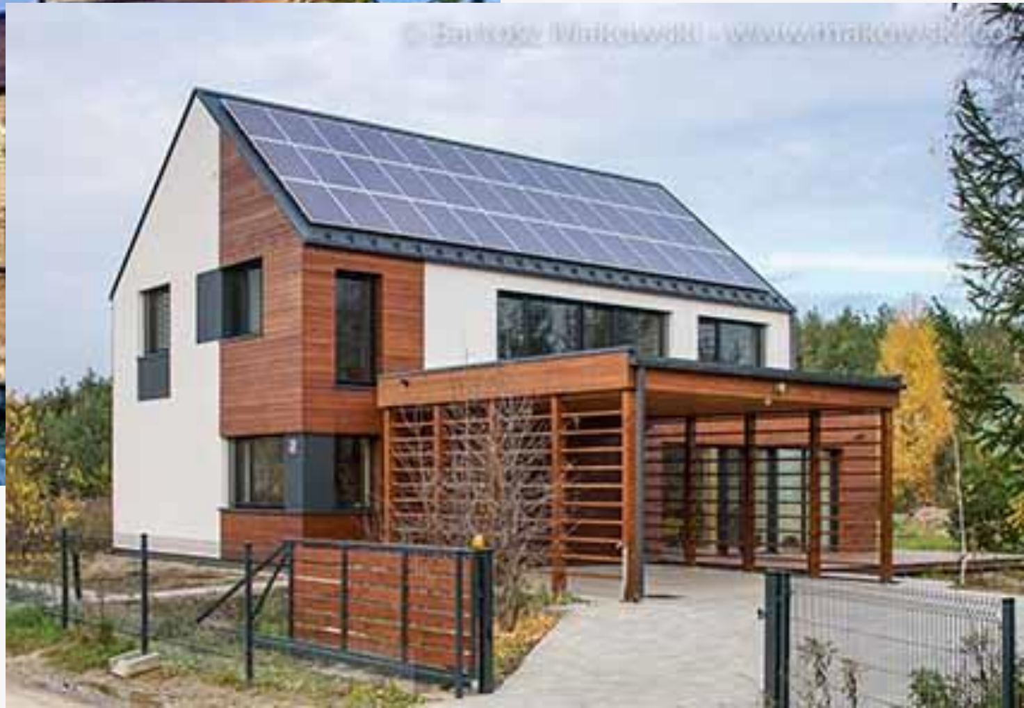
Dąbrowa Chotomska (Mazowieckie) Passivhaus Net Zero Energy timber construction
